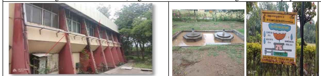
A Visual of roof top & surface rainwater harvesting structures
