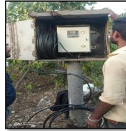
A Visual of Digital Water meter, Digital water level recorder along with telemetry service.
