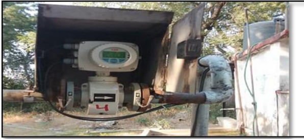
A Visual of Digital Water meter, Digital water level recorder along with telemetry service.
