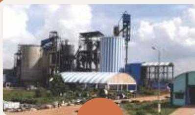
Grinding Unit at Cuttack
