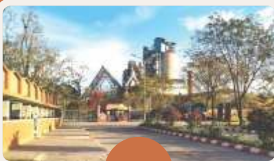
Integrated Unit at Udaipur
