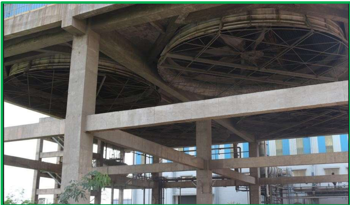
Air Cooled Condenser installed at Waste Heat Recovery
