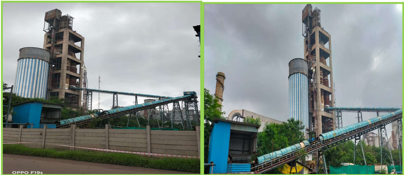
AFR System for Co- processing of Plastic & hazardous waste material
