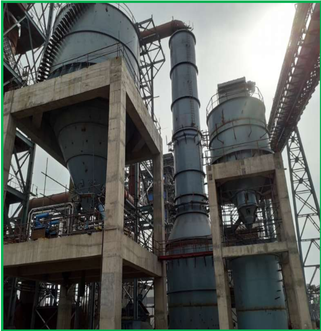
Flue Gas Desulphurization installed at Captive Power Plant
