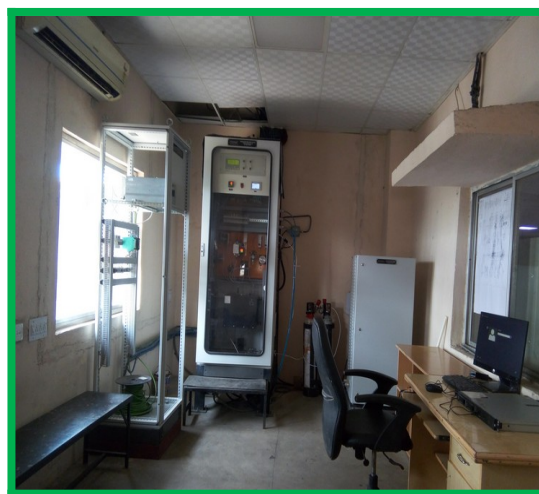
RABH CEMS and Opacity Meter installed at CPP stack and Server Room
