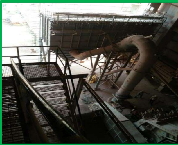
As a dust control measures we have installed Bag houses and Water sprinkling system over conveyor belts.
