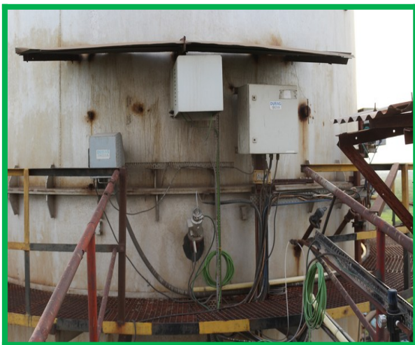
RABH CEMS and Opacity Meter installed at CPP stack and Server Room
