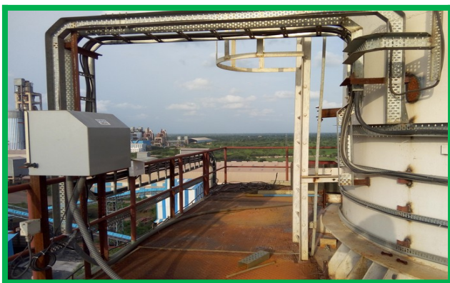
CPP CEMS and Opacity Meter installed at CPP stack and Server Room
