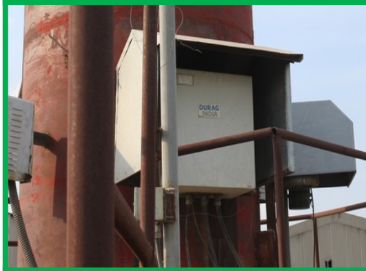
Cement Mill-2 Opacity meter
