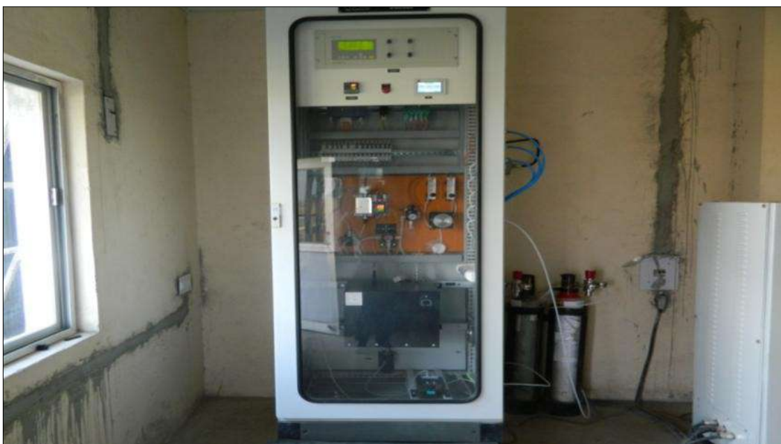
Continuous Emission Monitoring System For SO x , No x & CO Monitoring
