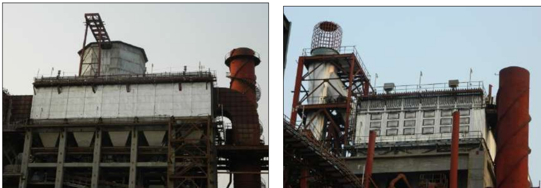
Slag mill and Coal mill Bag House
