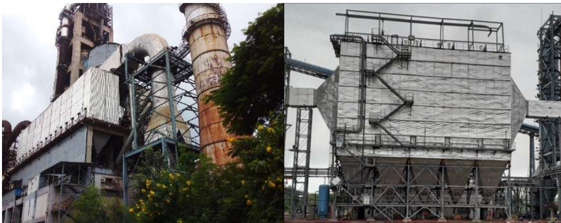
Reverse Air Bag House and Electrostatic Precipitator
