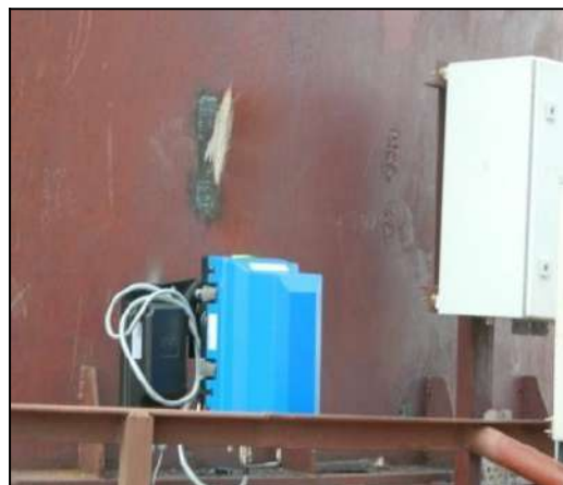
Opacity meters installed at all major stacks
