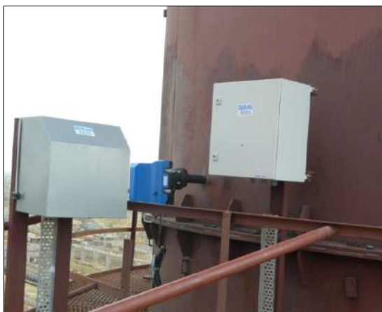
Opacity meters installed at all major stacks
