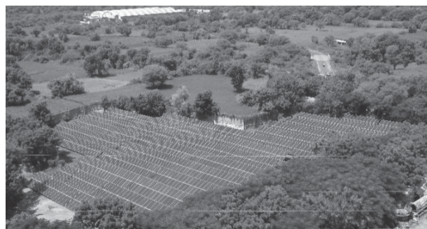
500 KW Solar Power Plant at Kalol, Gujarat
