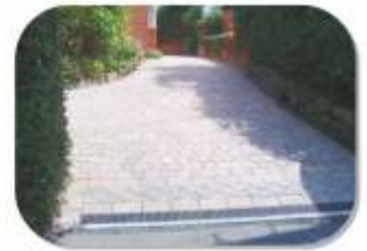
Residential & Commercial Driveways
