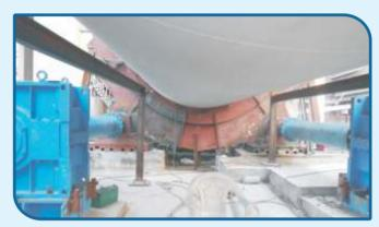
Hot Air Recirculation in line-1 IKN cooler installed as part of the Company's Power Saving Initiative
