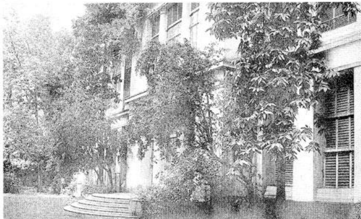
J K House on Kolkata's Alipore Road, from where the Singhanian family businesses were run until the 1970s
